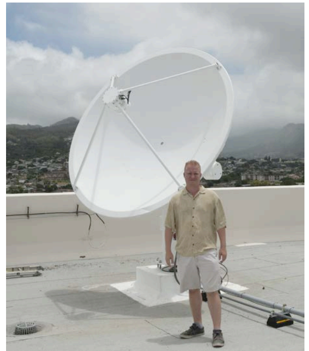
The satellite communication system is seen here on the roof of an HCC campus building. Roy Huff, foreground, is a post doctoral fellow at UH Manoa and oversaw the required rooftop engineering for the system. Courtesy: Steven Businger, UHM/SOEST.
