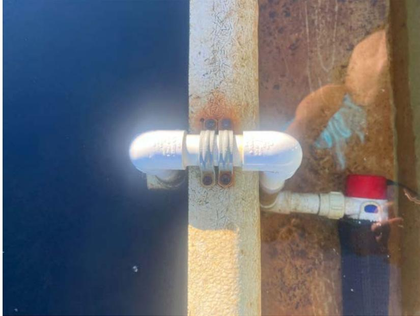
**Figure 22. Bilge pump and PVC pipe for water exiting the trough.**
