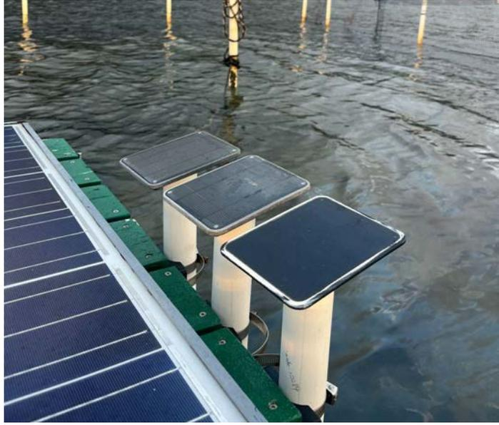
**Figure 10. Solar panels that power the sensors.**
