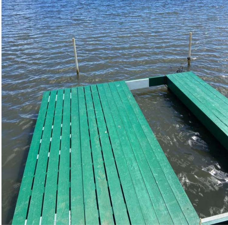
**Figure 21. Flooring on the FLUPSY, showing the 43-inch gap used for the trough and bins.**
