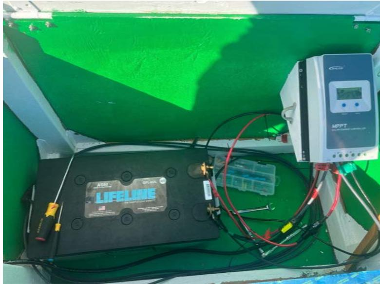
**Figure 24. FLUPSY battery and Solar Charge Controller.**
