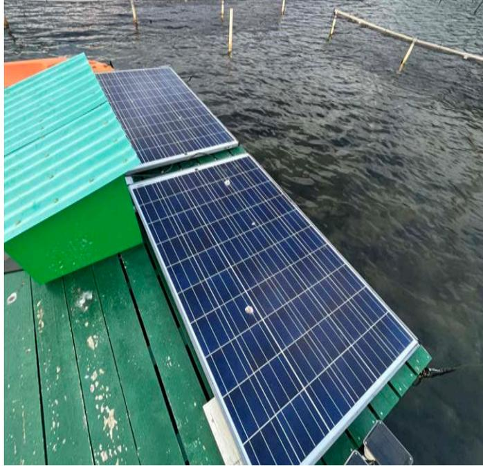
**Figure 26. Solar Panels on the FLUPSY.**
