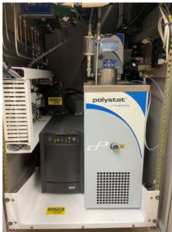
Figure 8: Polystat humidifier which was filled with deionized water to control relative humidity and dewpoint for the space in the reactor.
