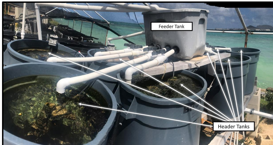
Figure 4: Close up of Feeder Tank and Header Tanks
