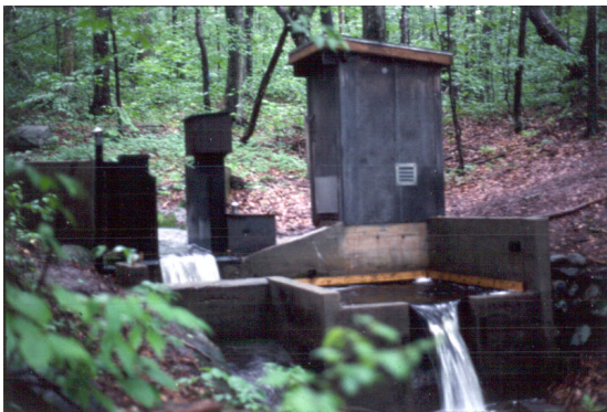
Example of a weir at Hubbard Brook:
