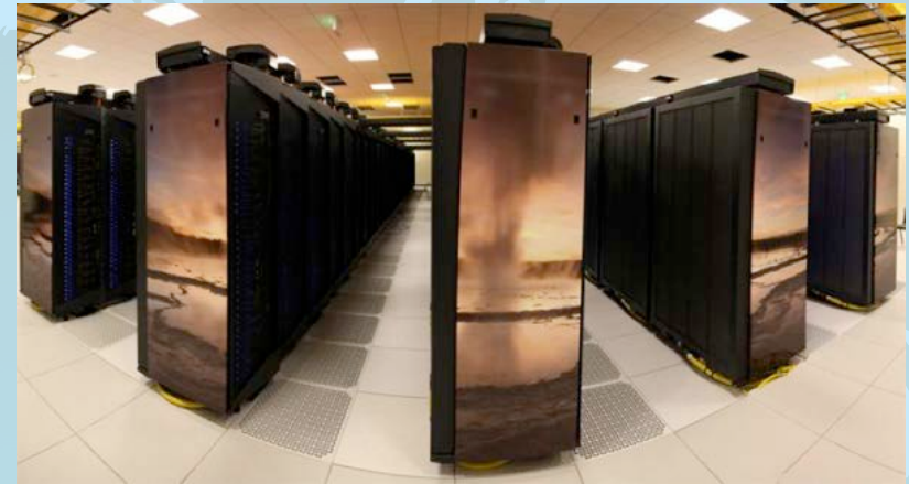
Yellowstone is an IBM iDataPlex supercomputer system, consisting of 149.2 terabytes of memory, 74,592 processor cores, and a peak computational rate of 1.6 petaflops.
