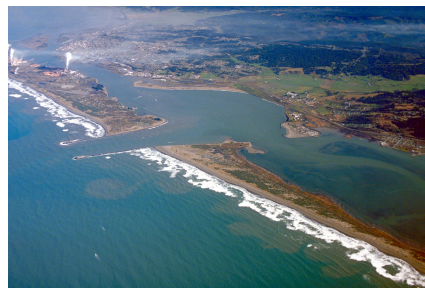
Jetties constructed of dolos at Humboldt Bay harbor
