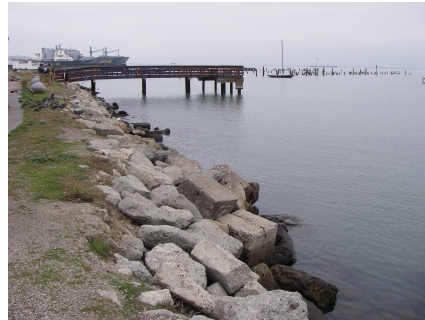
Riprap along San Francisco Bay
