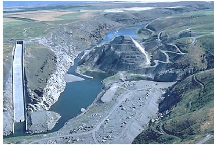
Teton Dam and reservoir, after failure
