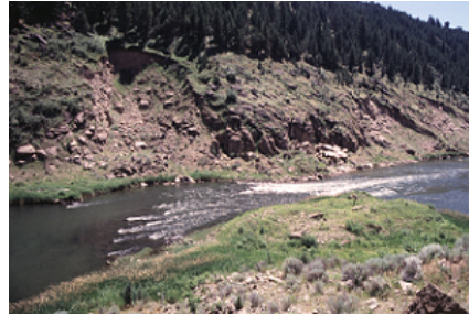
Landslide after loss of reservoir
