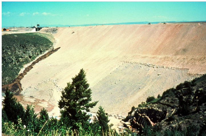
Note D-9 bulldozer heading down to upper leak. Another leak at toe.
