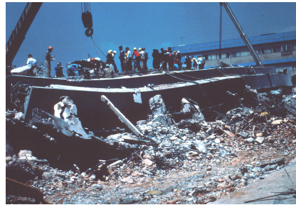
Collapsed General Hospital 1985 Mexico City earthquake
