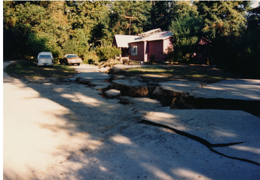
Fissure at head of a deep-seated slide, Summit Road
