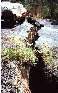
Crack in Hilina Pali Road
