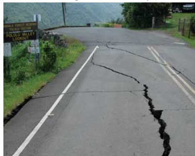
Road damage, Pololu Valley (Kahala)
