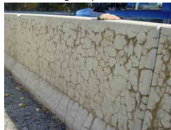
Cracks in a highway barrier from ASR
