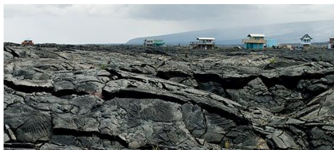
Fig. 11. The old Kalapana Gardens, which was buried under 40 to 60 feet of lava in 1990, is being replaced directly above by the rebuilt Kalapana Gardens. (Koning, 2018).
