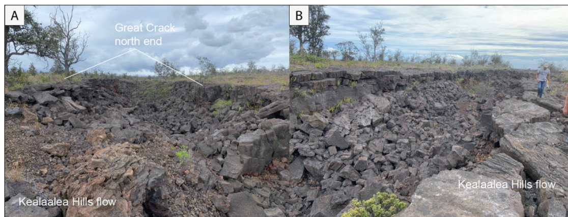
Fig. 16. Great Crack where it breaks the Kealaalea Hills lava flow – erupted less than 33 years prior - that shows no syn-eruptive widening or drain-back features. Also shows that the Great Crack is not as deep in the northern portion as it is down to the southwest.
