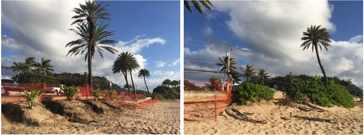
Figure 15. Native vegetation along the Sunset Beach bike path played a critical role in reducing scour and erosion, and maintaining beach sands in place along the upper berm (May 2017).
