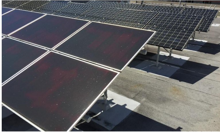
Figure 1 – Rooftop installation of the two tested PV technologies, micromorph tandem MHI (front) and polycrystalline KYO (back).
