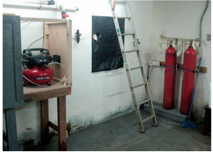
Figure 4. Compressed-air reservoir and CO 2 cylinder bank. Photo: Donald Bromhead
