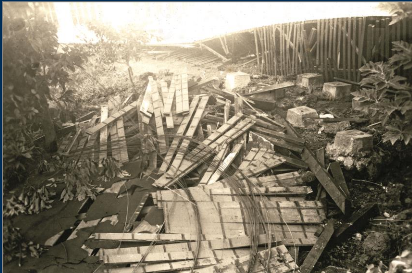
Collapsed water tank at Hōnaunau School in South Kona, Hawai'i. USGS photo.
