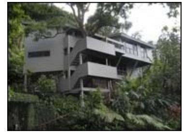
The Manoa Ecohouse, designed by architect Scott Wilson, is owned by Duane and Sarah Preble.
