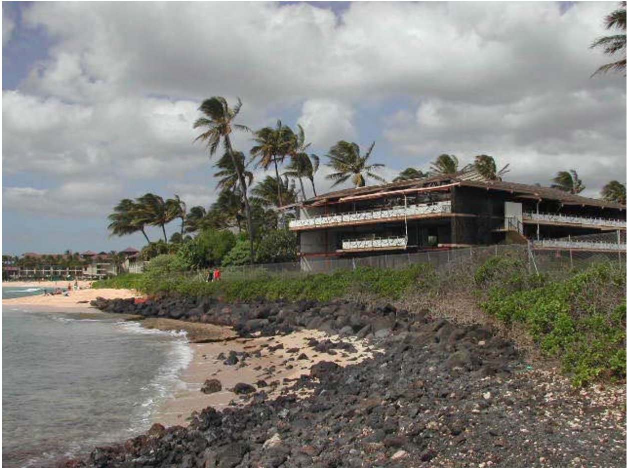
Hurricane Iniki storm surge damage, Poipu beach, Kauai. SJM 2/10/02.
