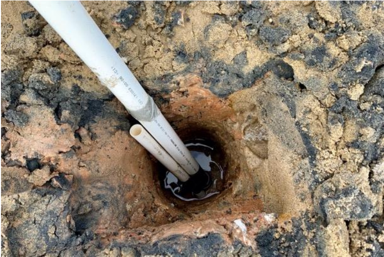
Fig S1.3. Example of a well dug during this study.
