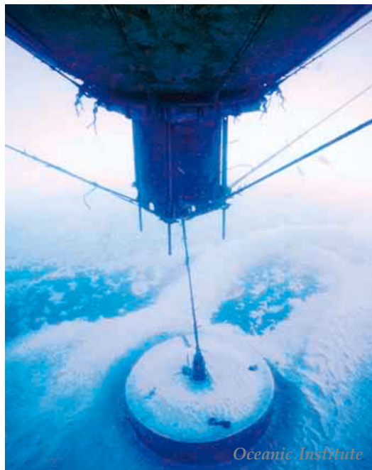
The HOARP experimental sea cage is submerged 40 feet below the surface and designed to withstand 25-foot waves. The cage acts as a fish aggregating device.
