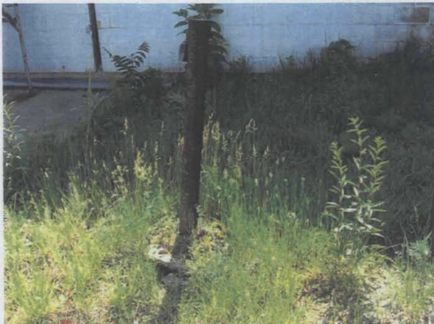
Photograph 1. Well NEP-104 (Note some heaving, but Jeffery Hamel reported that the bentonite seal was still intact)
