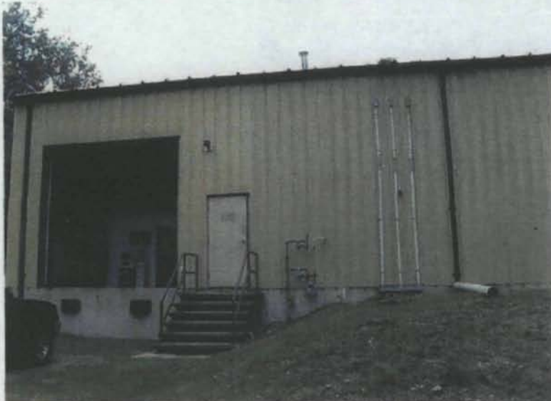
Treatment Facility Building.
