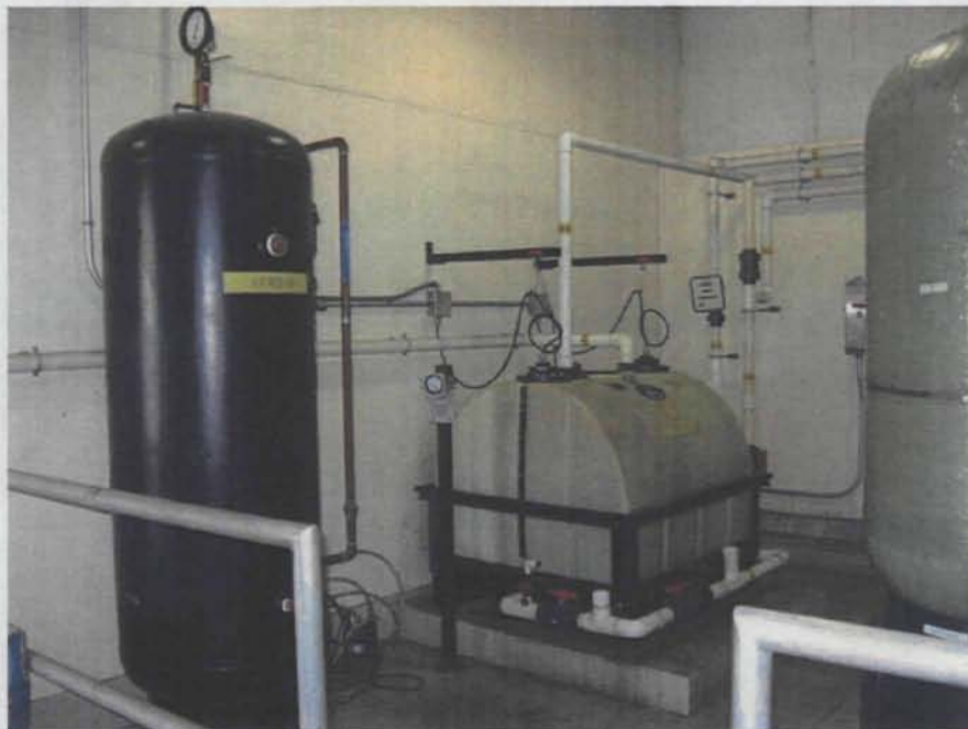
Photograph 2. Equalization Tank
